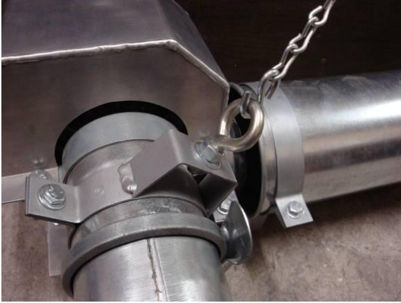
Photo 11: Small bracket attached at the correct angle
