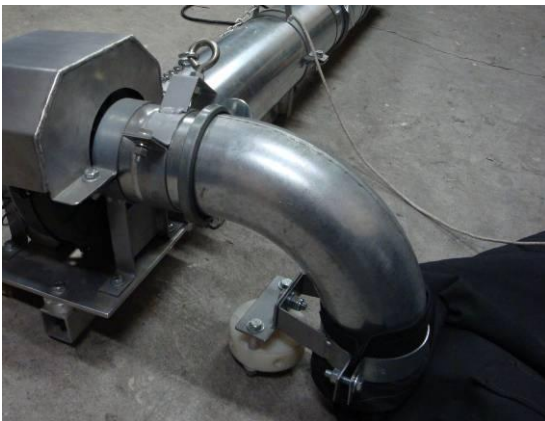
Photo 13: Canopy bracket attached to elbow with canopy collar clamped in between
