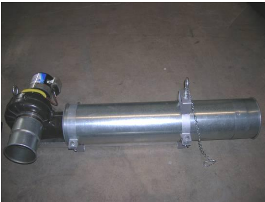
Photo 7: Second bracket installed on the right
